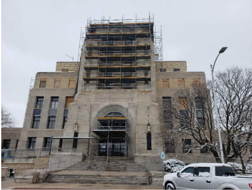
Figure 1. South elevation of the Reno County Courthouse.
