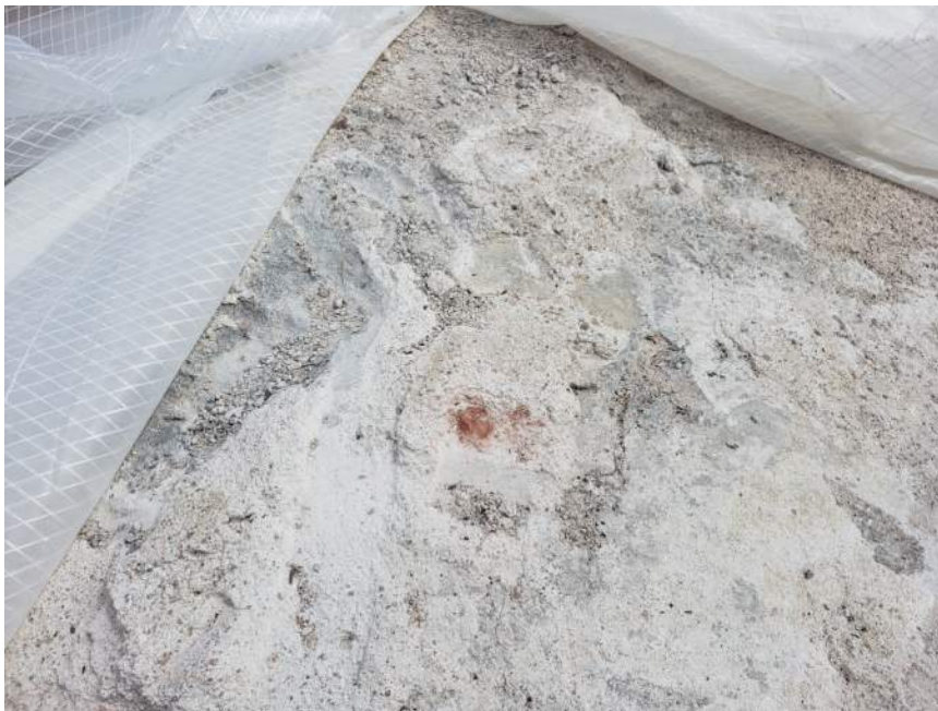
Figure 16. Southwest quadrant of the dome cap exposed.
