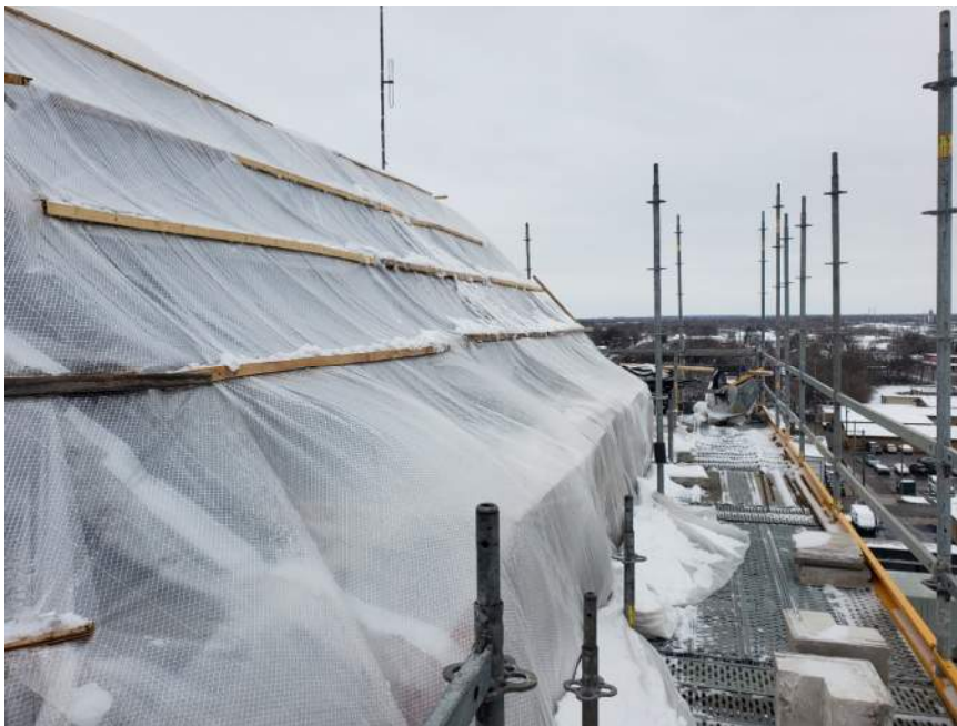
Figure 14. Tower dome covered in plastic.
