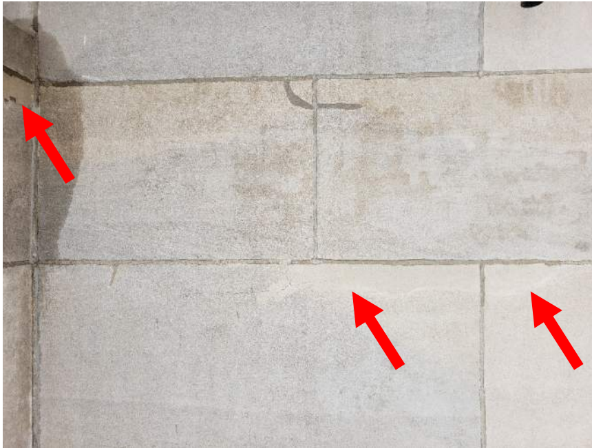
Figure 11. Locations of "half-moon" patch repairs (red arrows).
